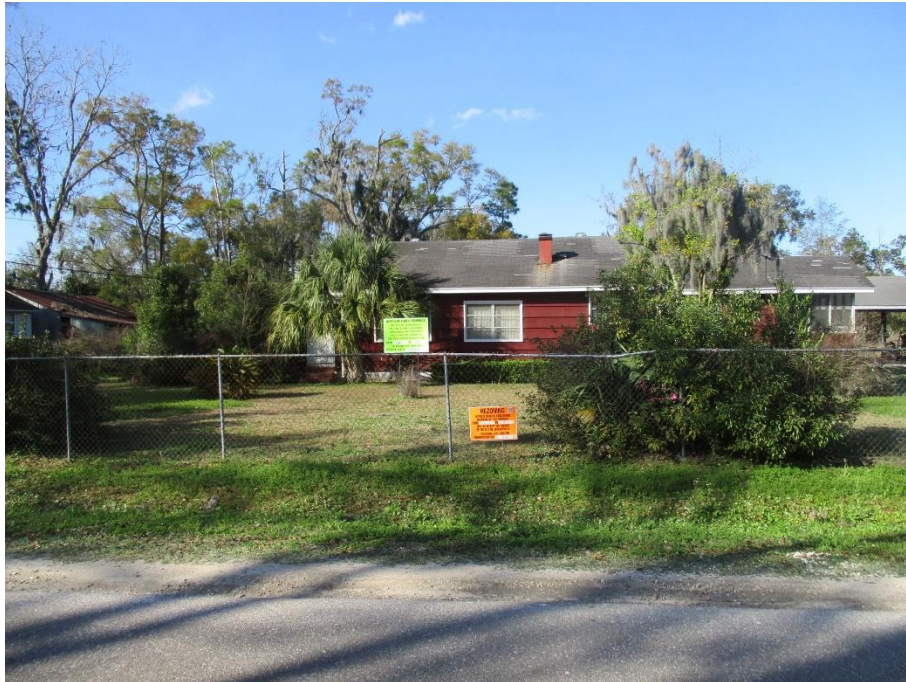
View of the subject property from Elizabeth Lane
